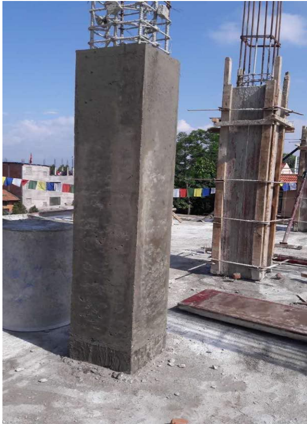
Columns On 4 th Floor
