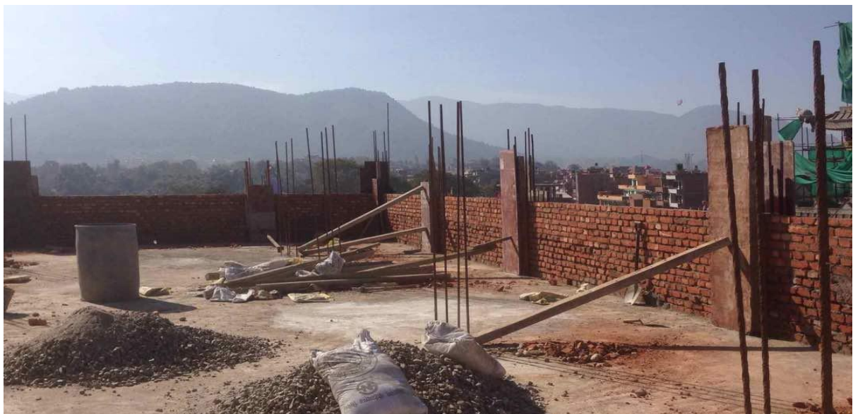
Brickwork on top floor
