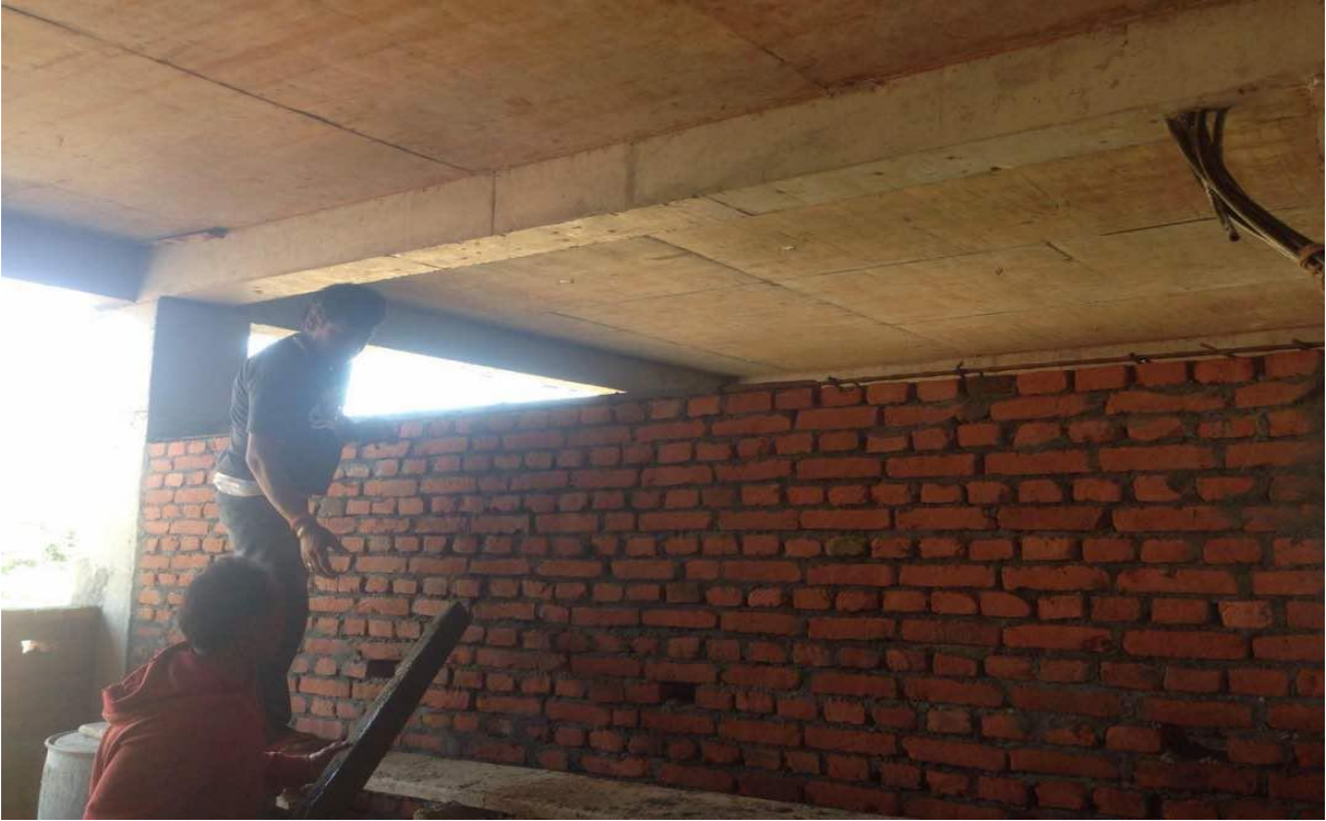
Brickwork On 3 rd Floor
